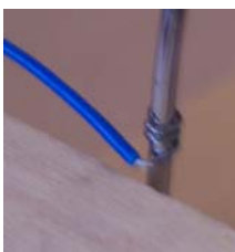
Image 2: The bare metal wire is wrapped tightly around a connection point and then taped in place.
